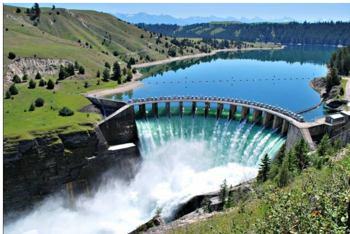
8 - HIDROELEKTRANE (HIDROELECTRIC POWER PLANT)
